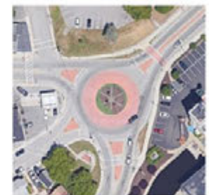
West Warwick Roundabout
