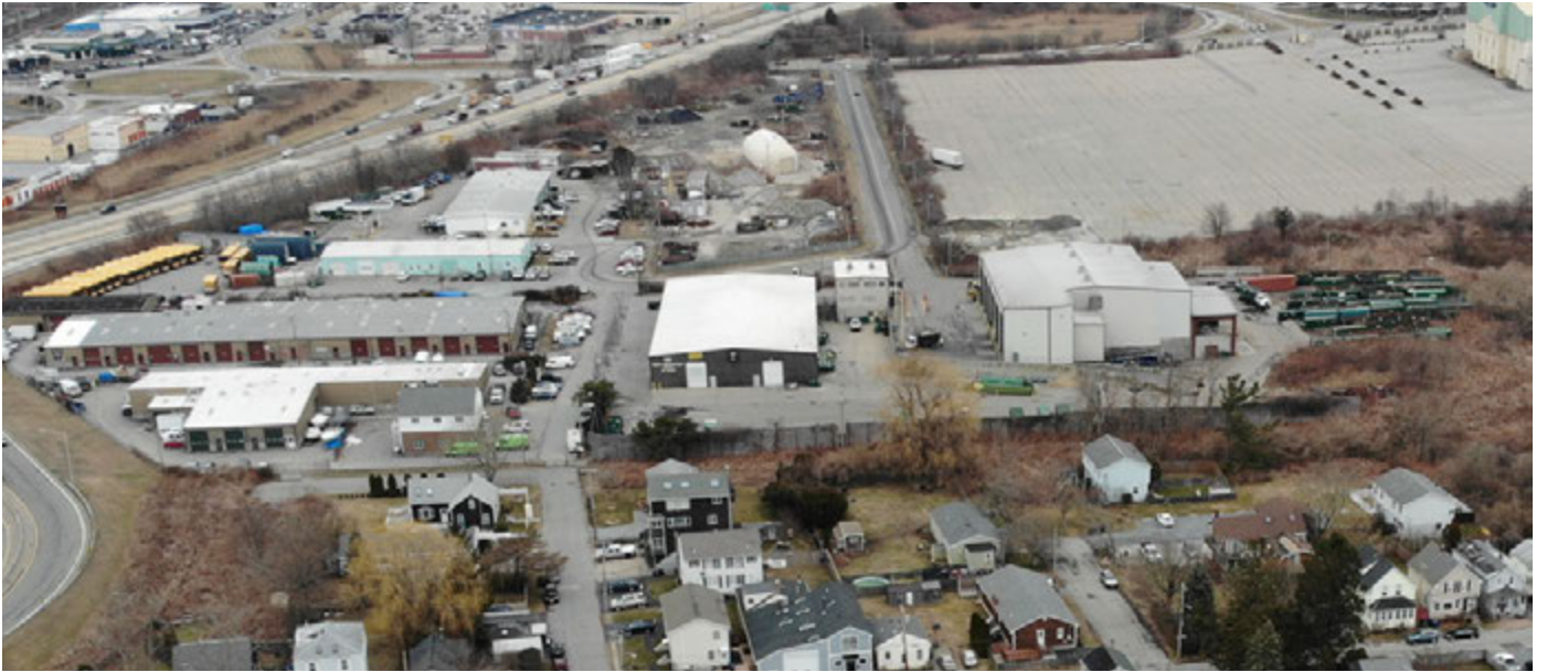
Aerial view of the Tradesmen's Center and Waste Transfer Station.
