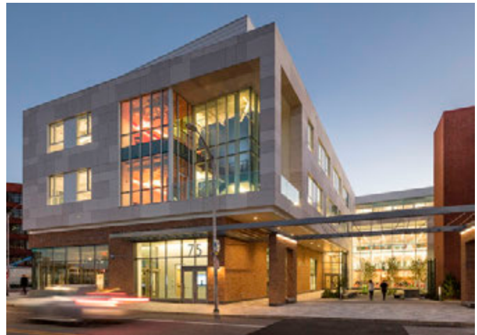
New office and technology buildings can create a more continuous street edge, as this example in Providence, RI shows.
